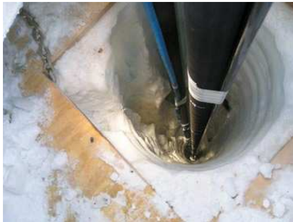
Figure 28: The hot water hose and support cables disappear down one of one of boreholes drilled into the Antarctic ice to construct the IceCube Neutrino Observatory. Photo: Jim Haugen [201]
