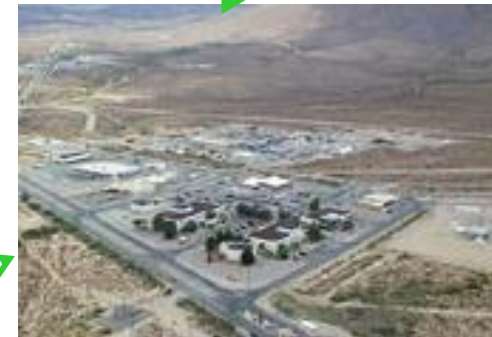
White Sands Ground Terminal, NM
