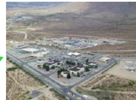
White Sands Ground Terminal, NM
