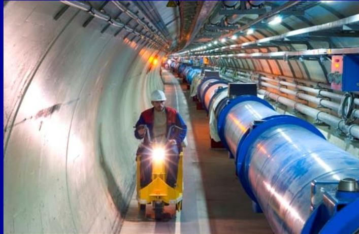
1.232 dipoli (14.3 m)  $8.3\text{ T @ }1,9\text{ K @ }12,84\text{ kA}$
