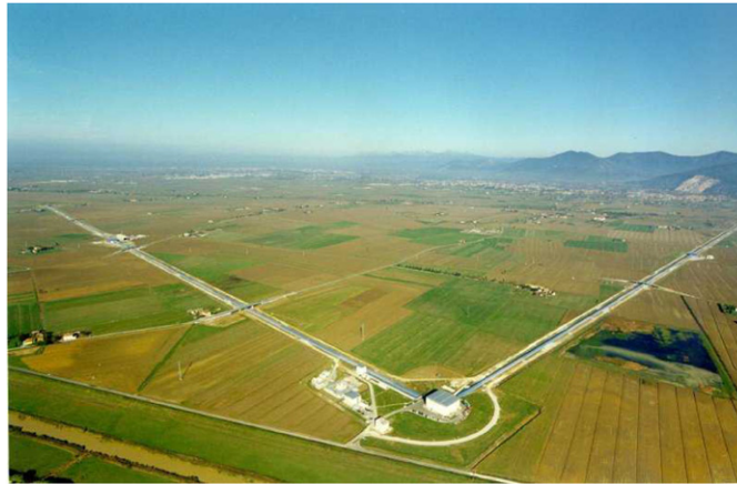
Figure 1. An aerial view of the Virgo gravitational wave detector. The detector Virgo is located in the countryside of Commune of Cascina, a few kilometres south of the city of Pisa, Tuscany.
